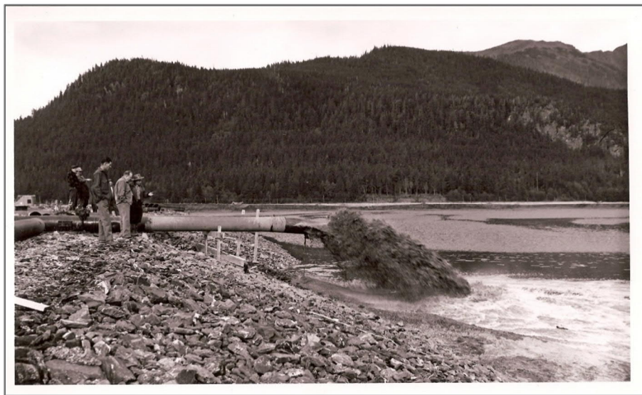
Figure 3-2: Construction of the Juneau International Airport
